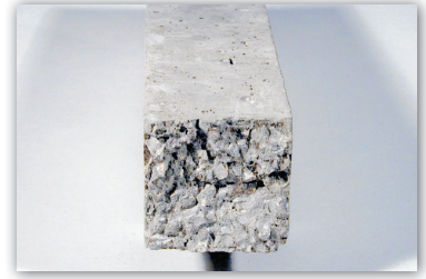
Ruptured Concrete Beam
